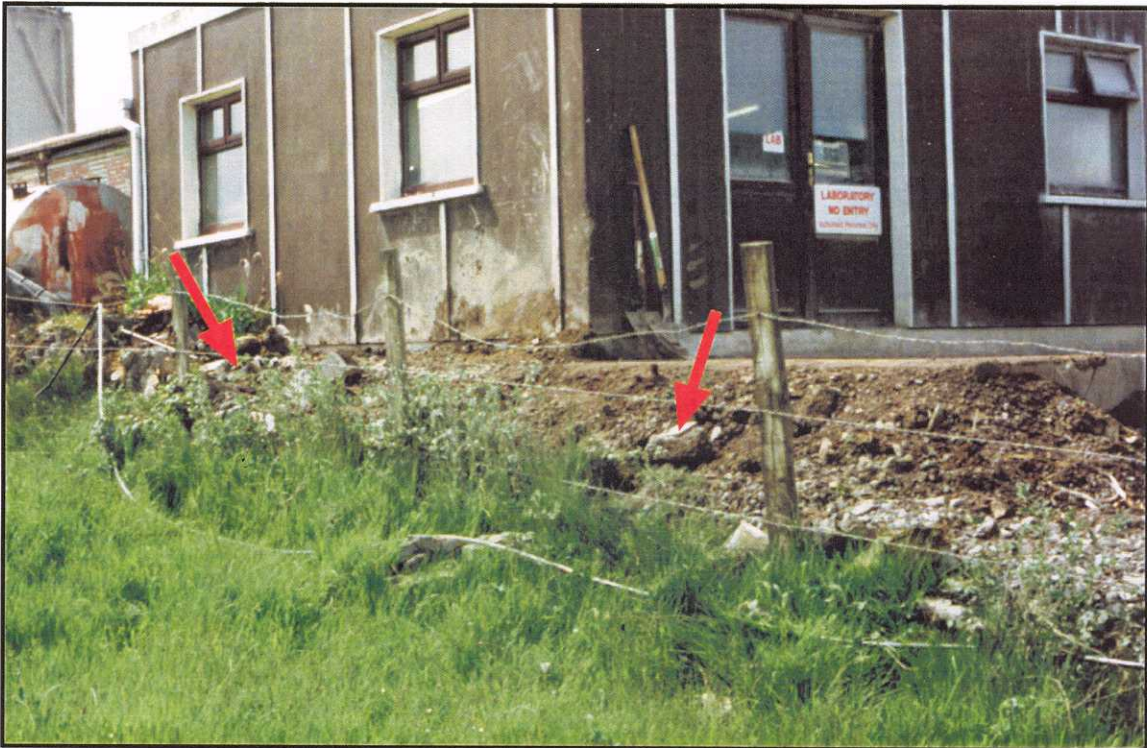
Boundary wall with quarry, removed without permission.
