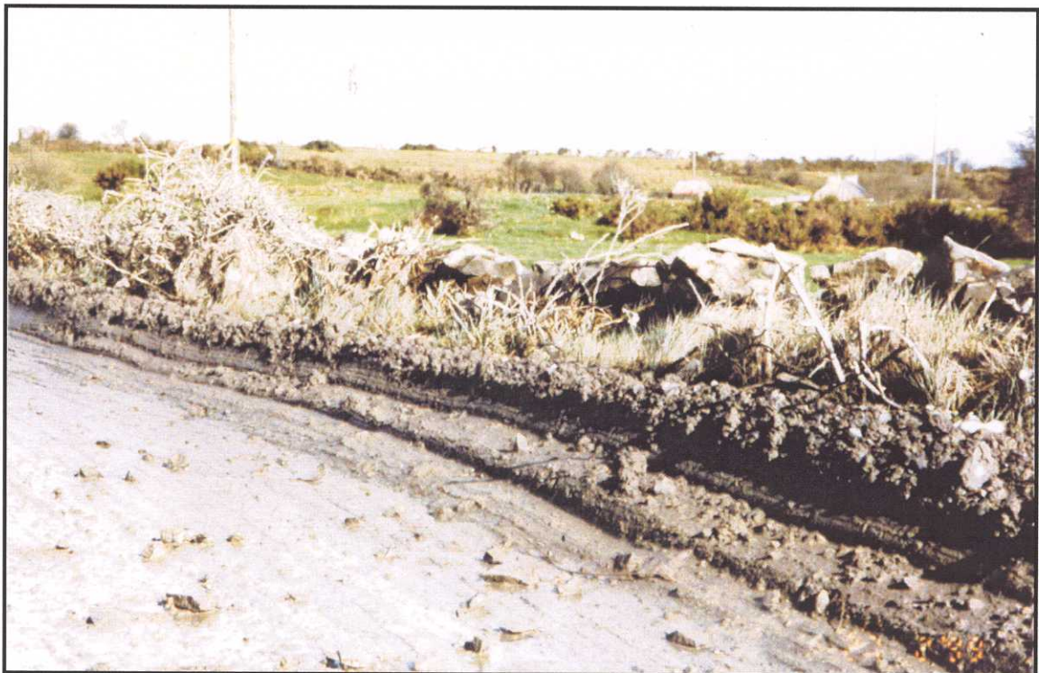
Level of access road almost equal with height of Gorman stone wall.
