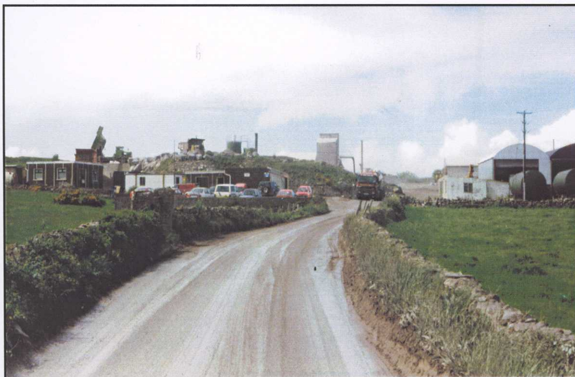
No mitigation measures for visual impact / dust emissions.
