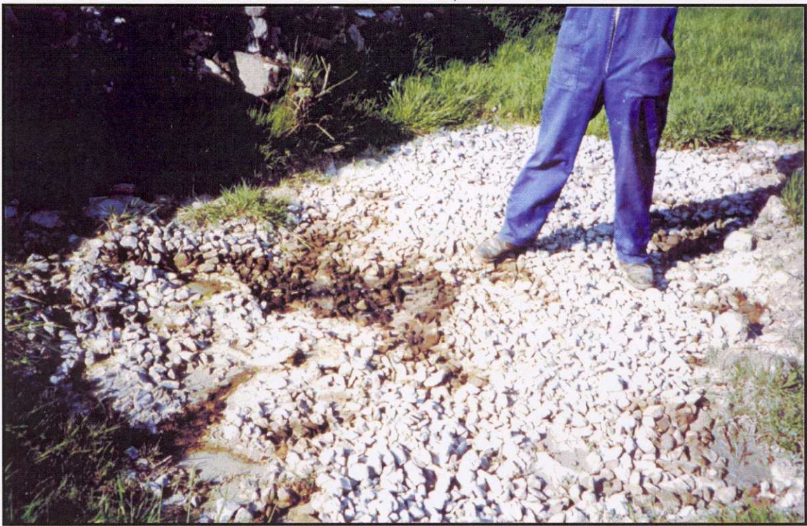
Stained soakway area from Mc Caffreys surface run-off.
