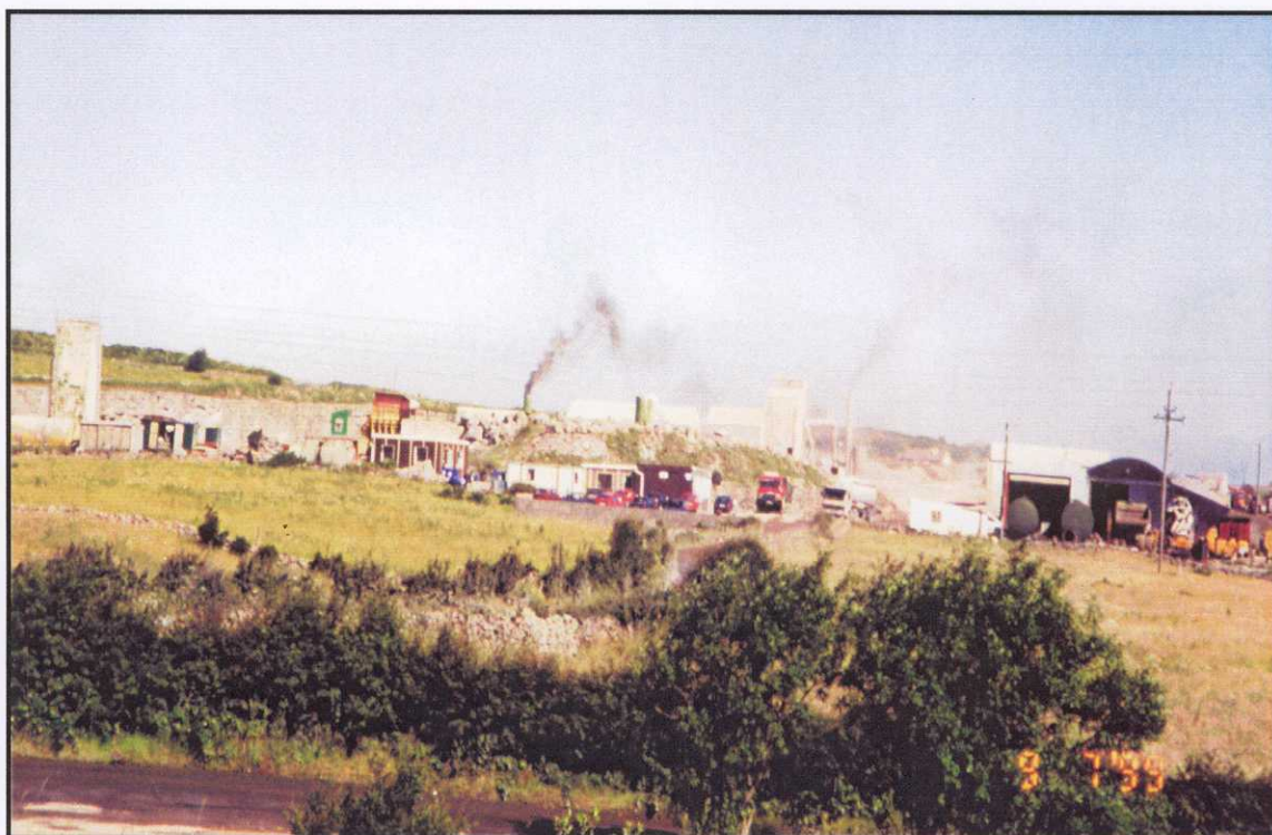
Air discharges from asphalt plants.
