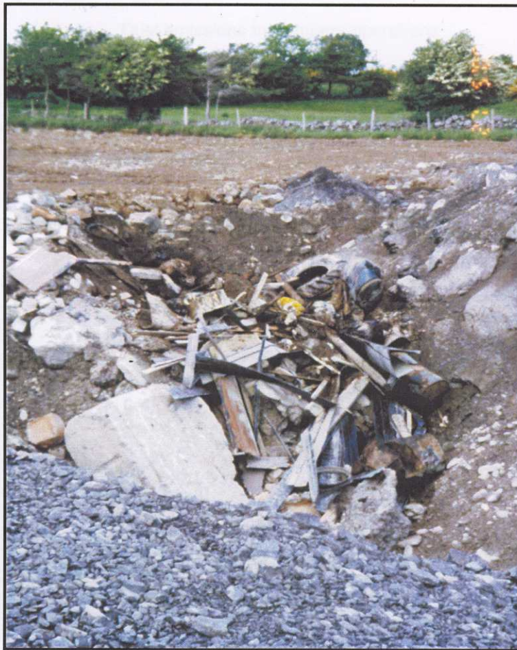
Quarry No. 3. (Partly backfilled with scrap metal/drums).
