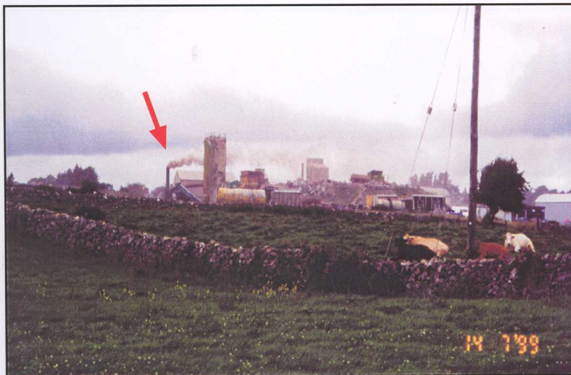
Air discharges from asphalt plants.
