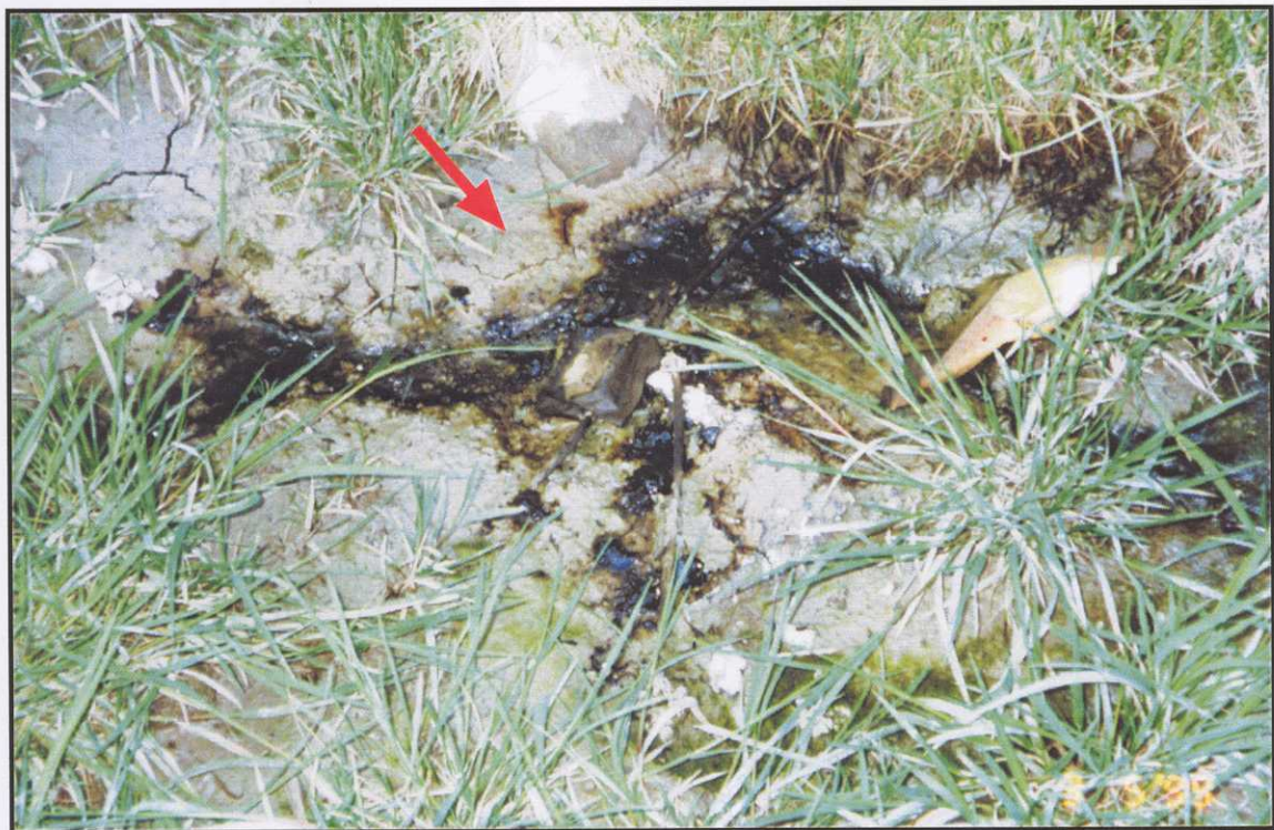
Bitumen residues that have flowed into the Gorman land.
