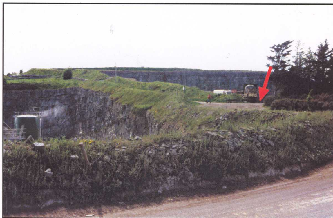
Public road running between unprotected cliff faces to quarries No. 1 and No. 2.
