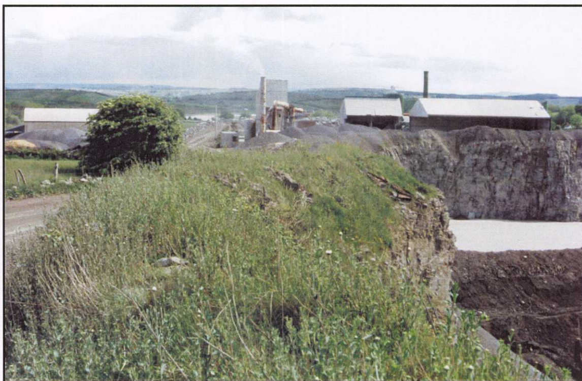
Unprotected cliff face to quarry No. 1 including tailings pond.
