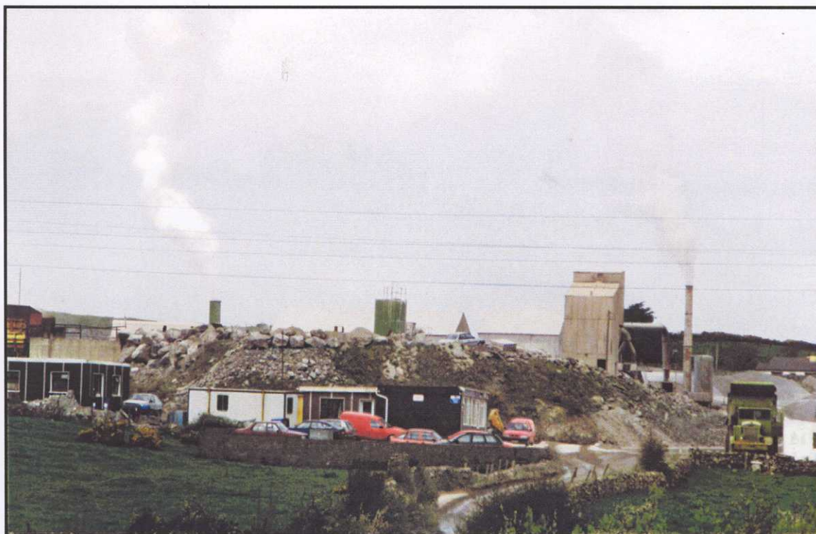
Air discharges from asphalt plants.
